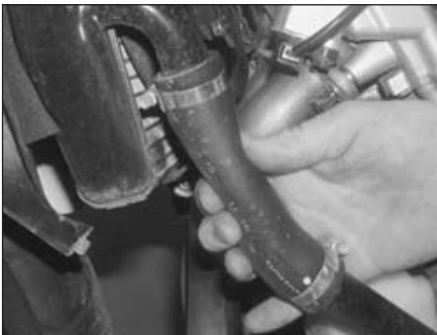
12.2 Check all the coolant hoses as described
