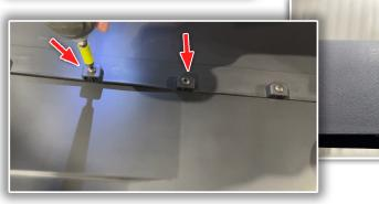
USE THE SELF TAPPING SCREWS PROVIDED IN YOUR KIT TO FIX THE FRONT AND REAR PIECES OF THE ROOF TOGETHER AS SHOWN IN THE IMAGE TO THE LEFT.
